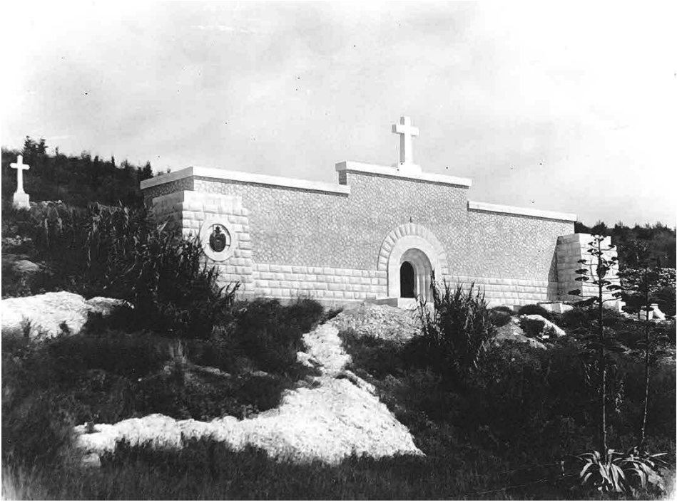
Picture 4: The ossuary during construction. Archives of Yugoslavia
